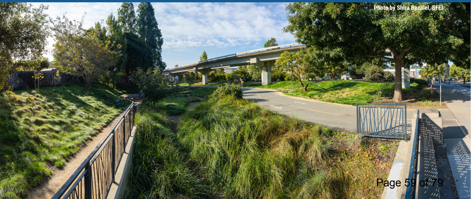
Below, rain garden in El Cerrito by BART tracks
