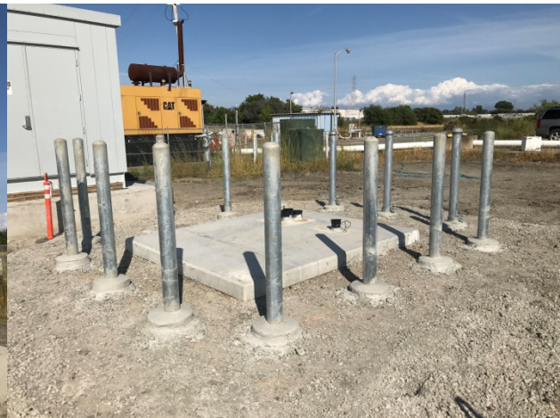
Transformer Pad Bollards
