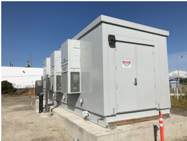
MCC Building Air Conditioning Units
