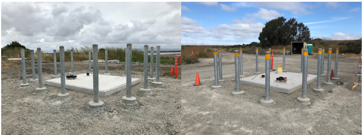
Transformer Pad Bollards - Before
