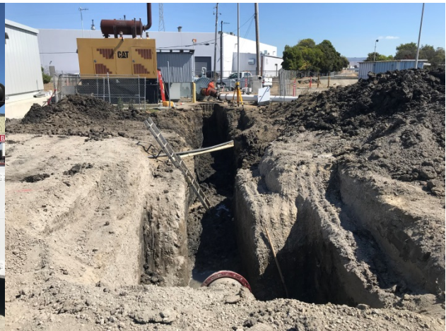
HDPE Pond Diversion Piping
