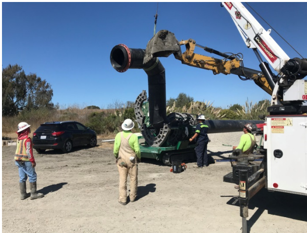
HDPE Pond Diversion Piping
