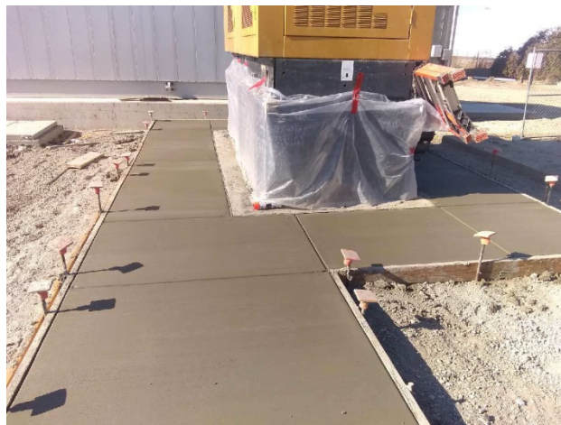
New Concrete Slab Around Generator
