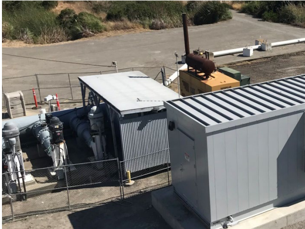
Before Old MCC Demolition
