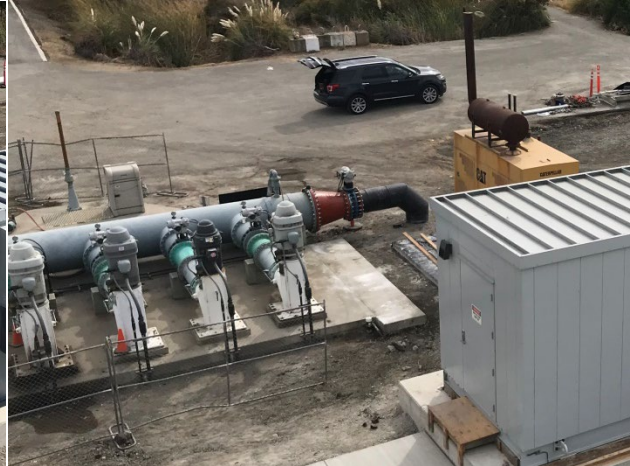
After Old MCC Demolition
