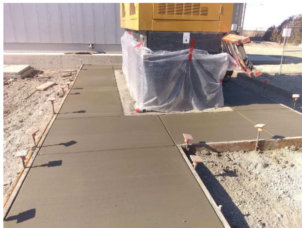
New Concrete Slab Around Generator
