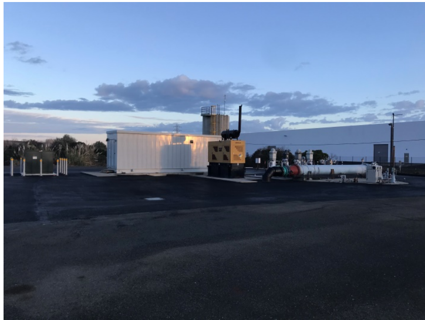
New HEPS Pavement
