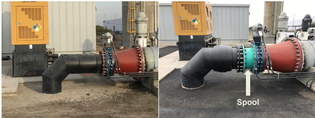
Before 24-Inch Steel Spool
