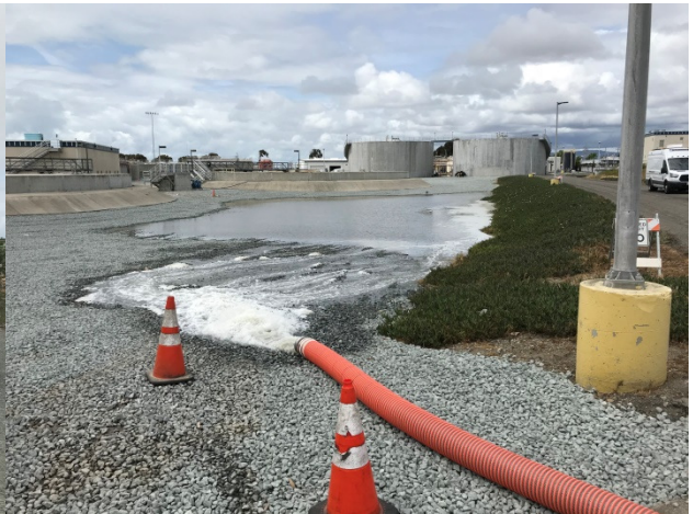
Pumping From Leak Area Back To The OLSD Plant
