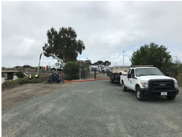
Pumping From Leak Area Back To The OLSD Plant
