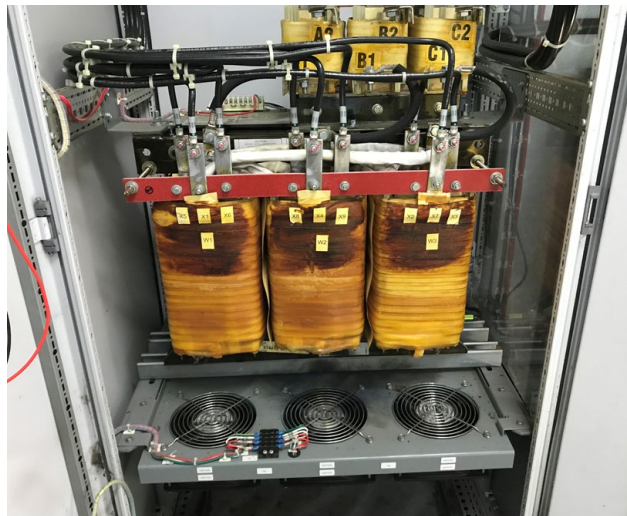
Effluent Pump No. 2 VFD Transformer
