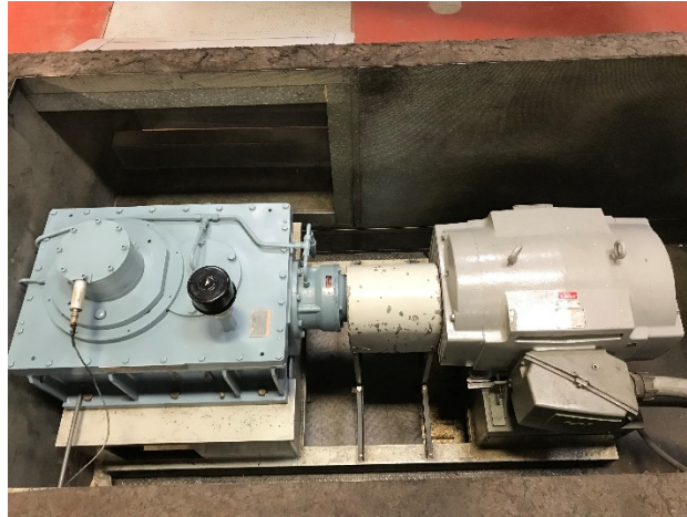
OLEPS No. 1 Effluent Pump Right Angle Gear Drive & Motor
