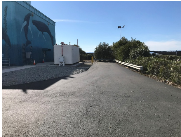
New Asphalt Behind OLEPS
