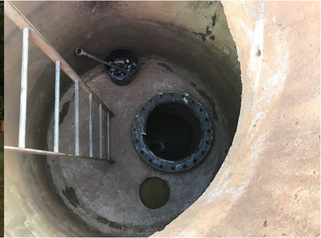
Inside Manhole Before Force Main Entry
