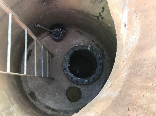
Inside Manhole Before Force Main Entry
