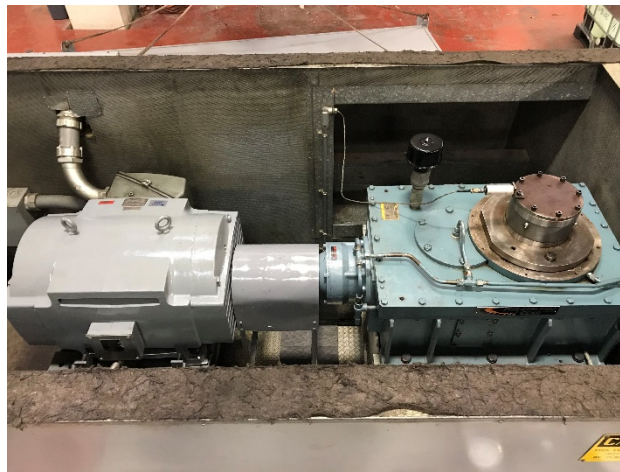
OLEPS Effluent Pump No. 4 Right Angle Gear Drive & Motor
