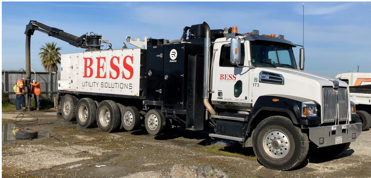
Vactor truck potholing the EBDA force main
