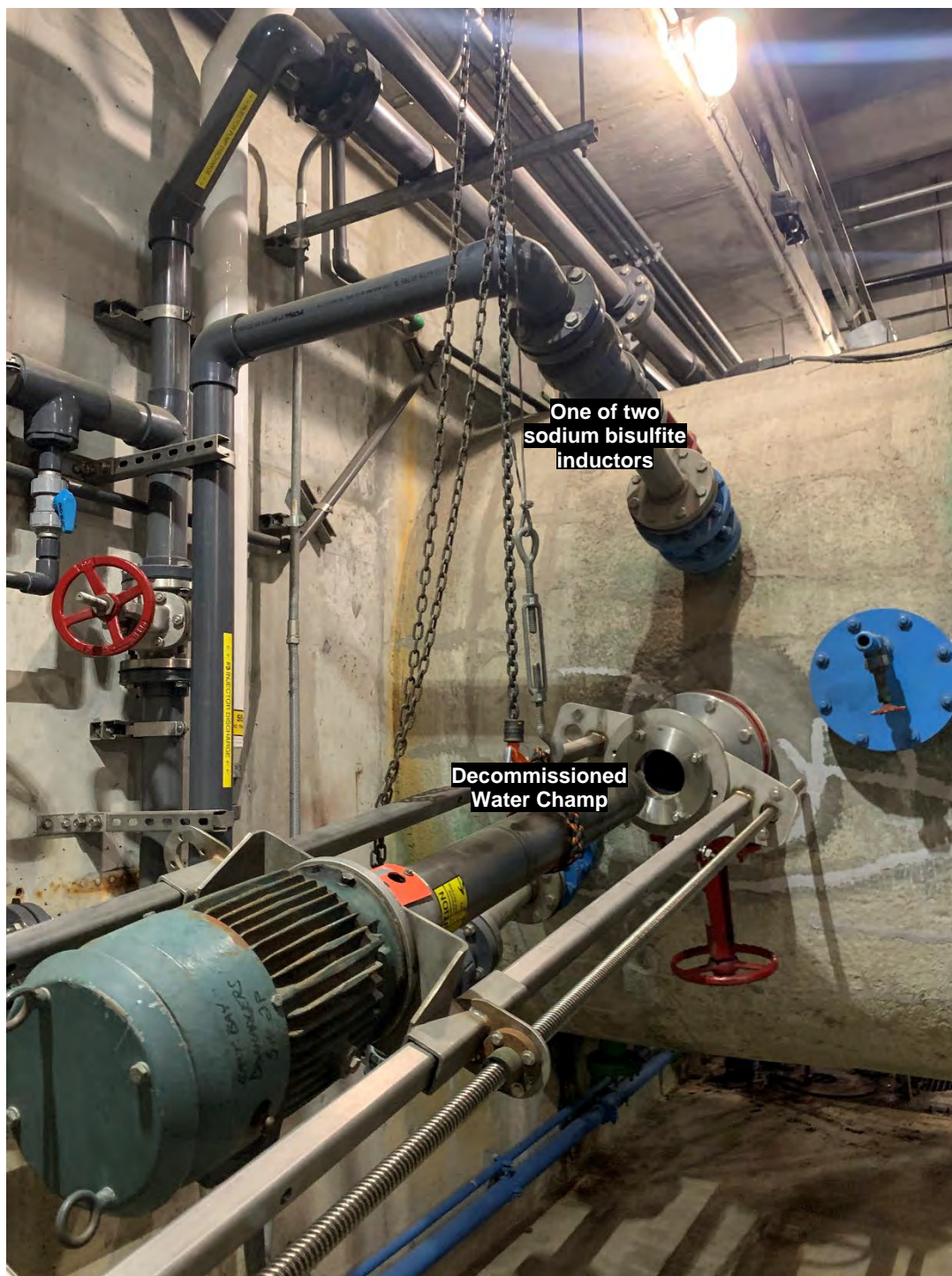
Figure 16. Sodium bisulfite is injected into effluent pipeline by two inductors immediately proceeding the convergence of the two influenced force mains. The decommissioned chemical mixer, or Water Champ, used to be EBDA's primary method of dechlorinating its effluent.
