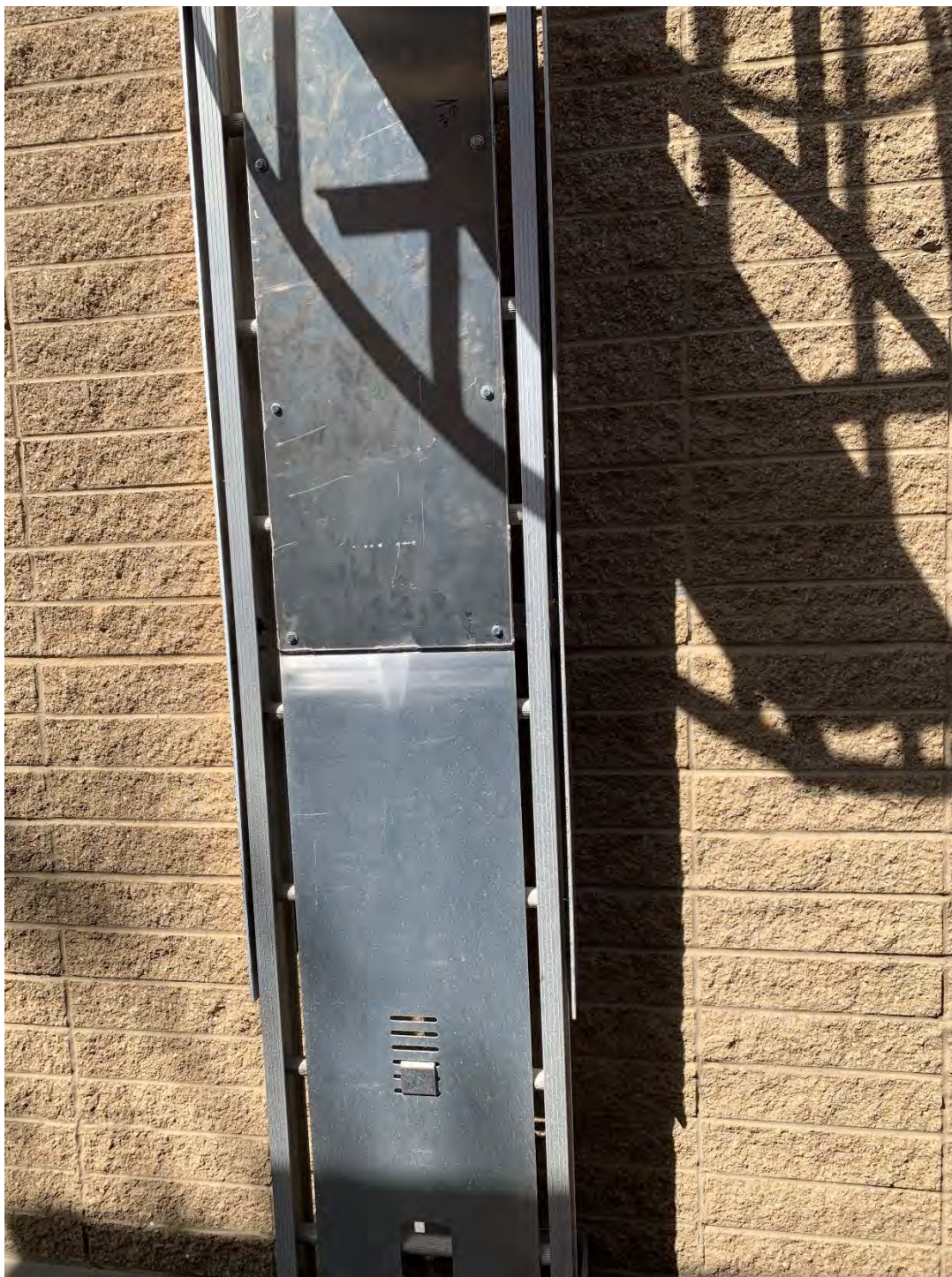
Figure 18. EBDA recently installed a metal ladder guard to prevent people from climbing to the roof of the sodium bisulfite storage building after hours.
