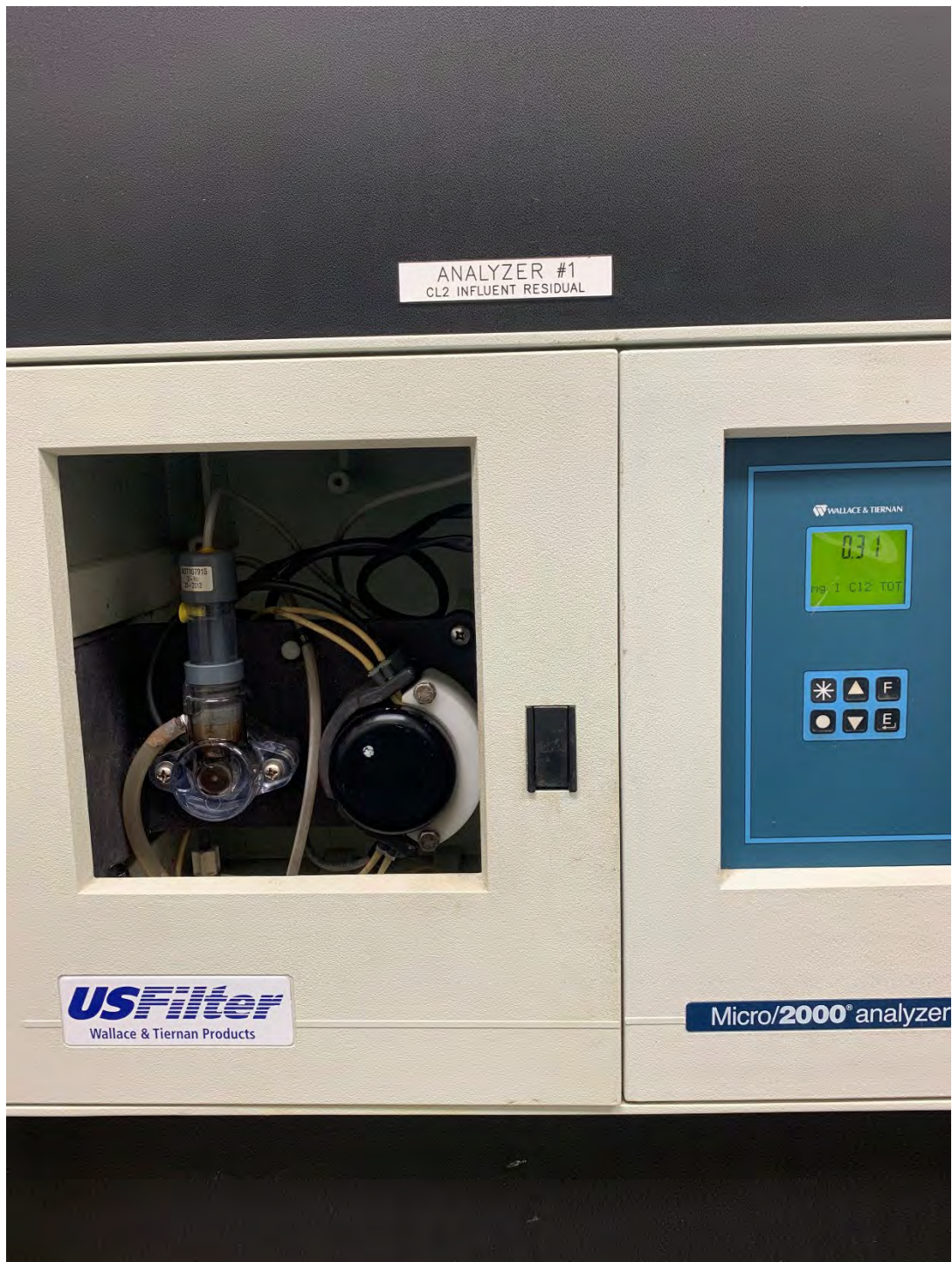
Figure 5. The influent chlorine analyzer read 0.31 mg/L at the time of the inspection.
