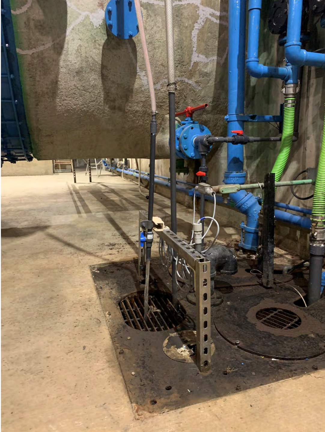
Figure 17. The bacteria sampling location just precedes the addition of sodium bisulfite.
