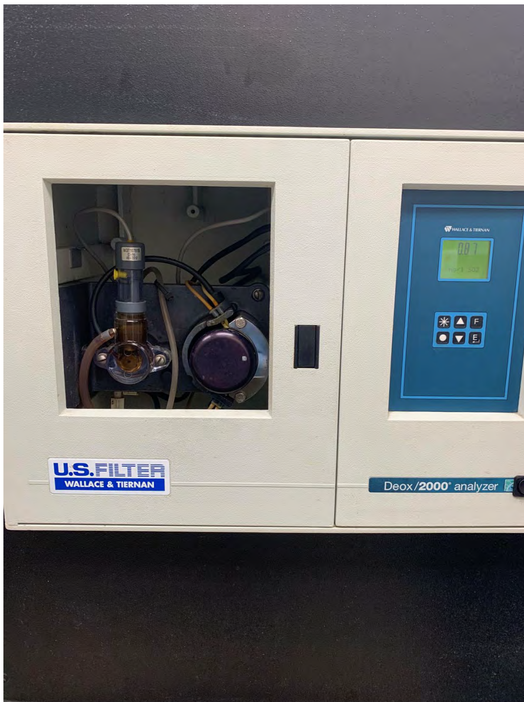
Figure 7. The effluent sodium bisulfite analyzer read 0.87 mg/L at the time of the inspection.
