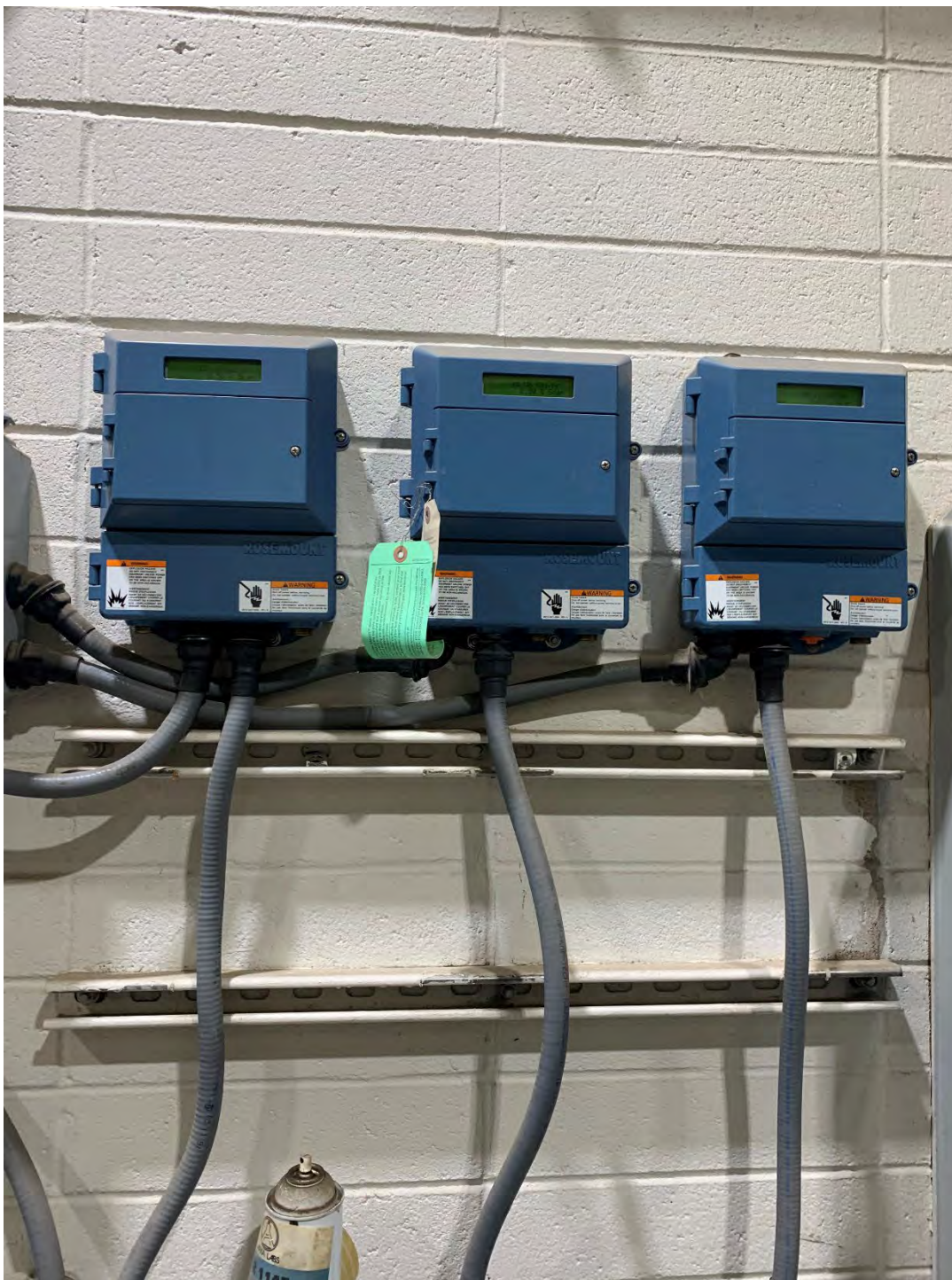
Figure 13. The three sodium bisulfite flow meters. One was online at the time of the inspection, consistent with the one sodium bisulfite pump that was also online.
