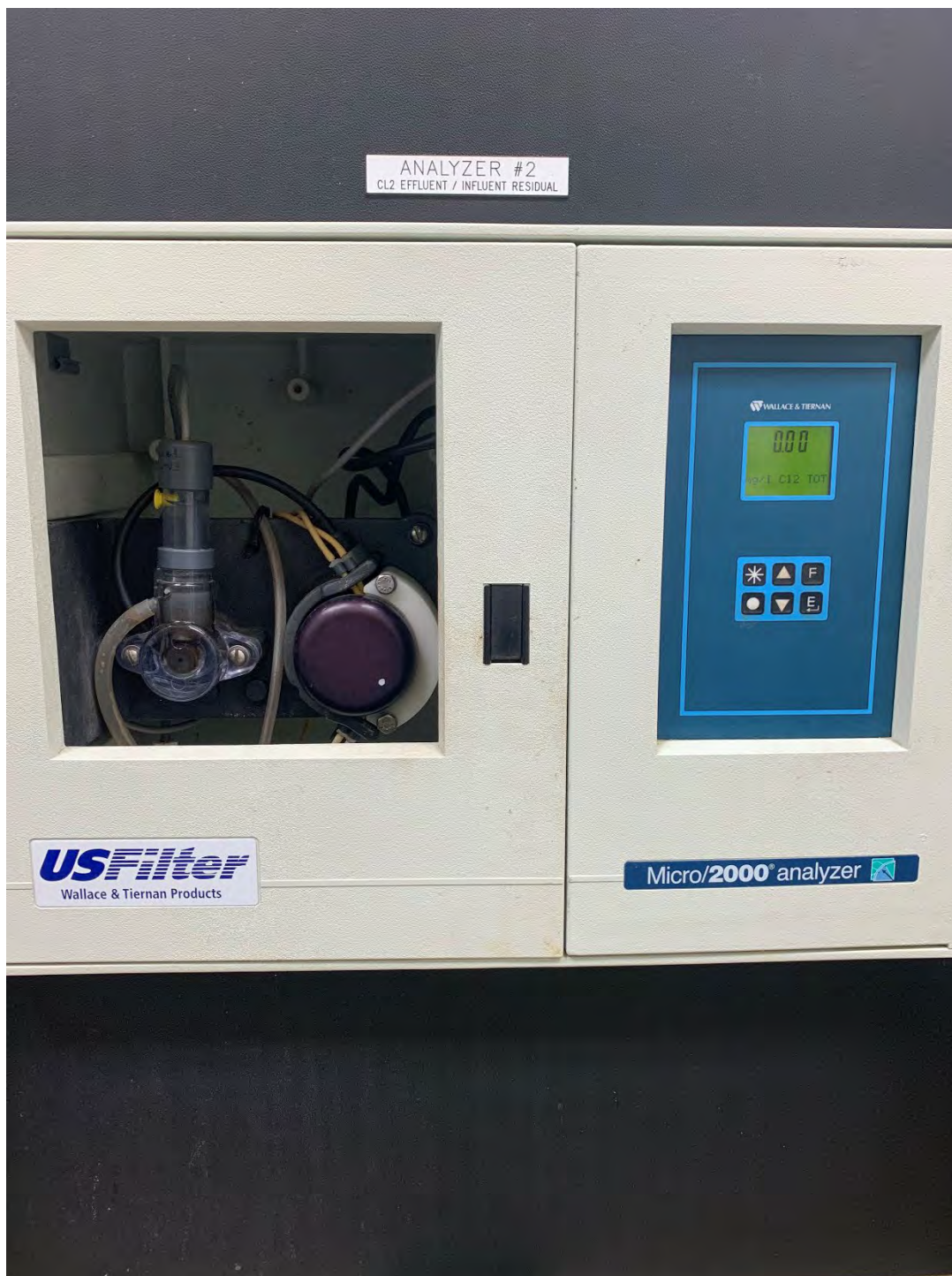
Figure 6. The effluent chlorine analyzer read 0.0 mg/L at the time of the inspection.
