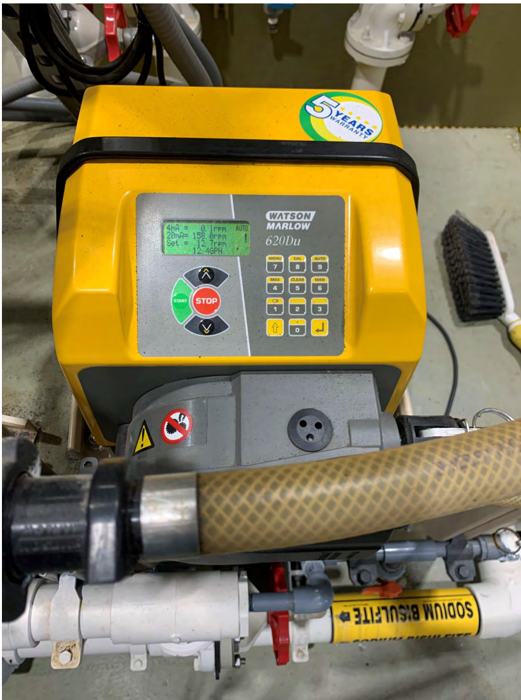
Figure 11. One of the three sodium bisulfite pumps. EBDA keeps one online with two as backups and rotates between the three every week.
