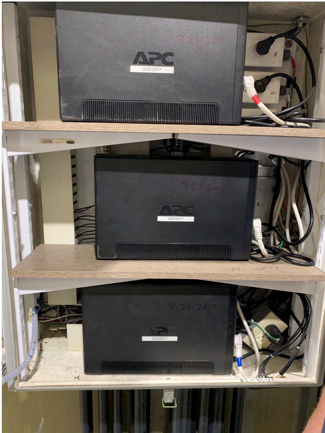
Figure 14. The three uninterruptible power supply boxes support the Facility's programmable logic controller during a power outage. EBDA plans to replace these boxes with new ones after July 1.
