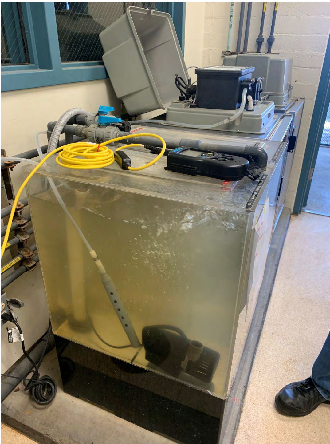
Figure 3. EBDA's sample holding tank is located in the control room, which contains dechlorinated effluent. At the time of the inspection, EBDA was evaluating dissolved oxygen concentrations in the discharge to determine how it might affect corrosion in the force mains once EBDA begins accepting brine.
