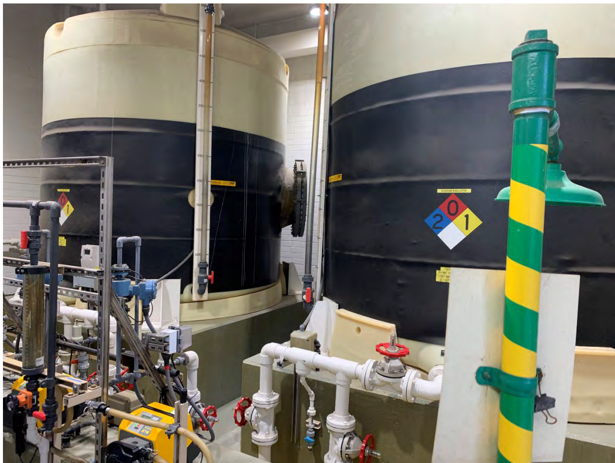
Figure 10. The Facility's sodium bisulfite storage building contained two, 6,000-gallon tanks of sodium bisulfite.
