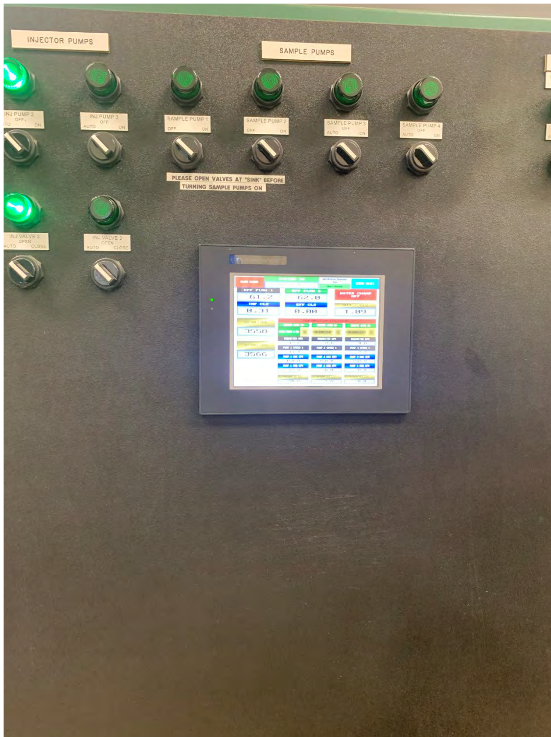
Figure 4. EBDA's programmable logic controller displays a screen of live pump operations at the Facility.
