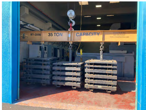
OLEPS Overhead Crane Quadrennial Load Testing
