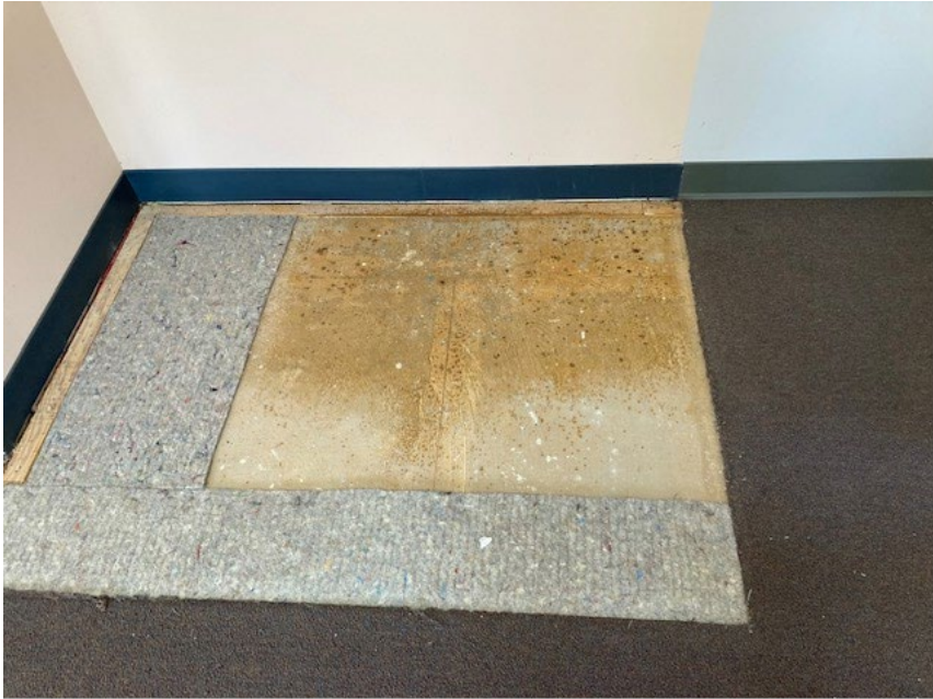
Mold Identified in the Floor under the Plan Drawers
