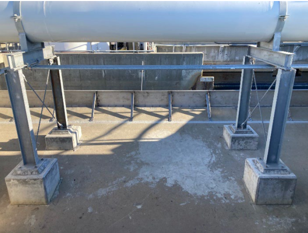
New Stainless-Steel Weir & Expansion Joint
