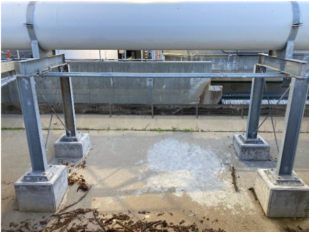
Old Lumber Weir & Expansion Joint
