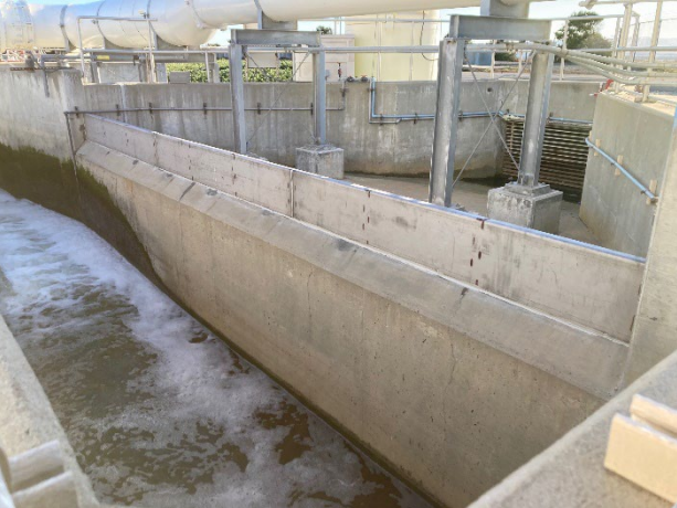
New Stainless-Steel Emergency Outfall Weir
