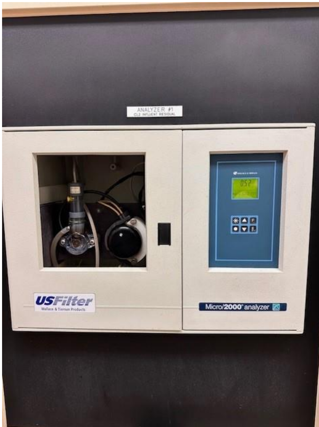
Figure 3. The influent chlorine analyzer read 0.52 mg/L at the time of the inspection.
