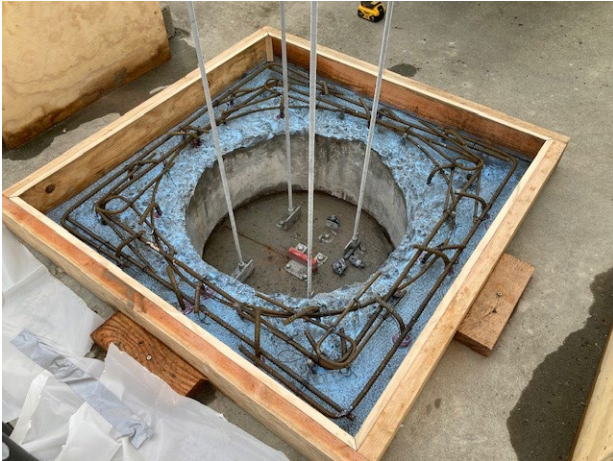
New Pump Base Rebar
