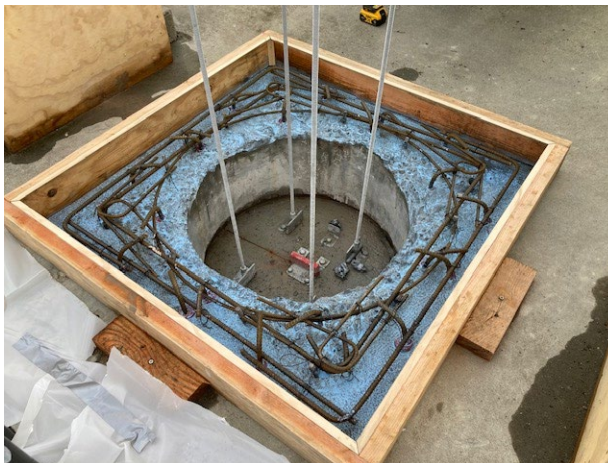
New Pump Base Rebar
