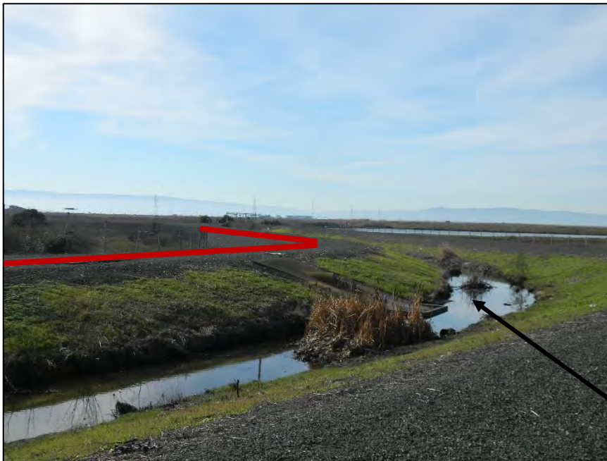
Photo 2 – View of drainage channel from railroad spur looking southwest. This channel was built after the EBDA pipeline, most likely resulting in locally reduced cover on the 60-inch RCP force main.
