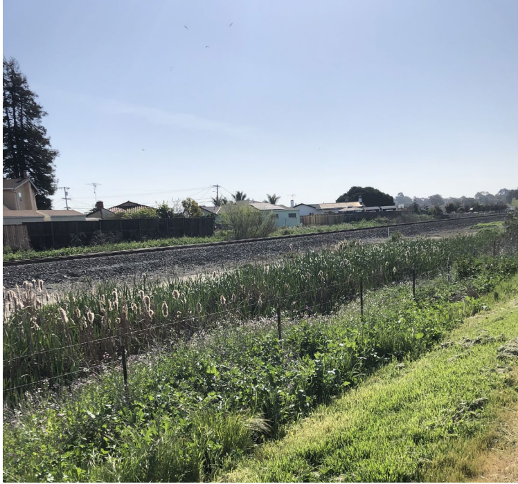
EBDA First Mile Horizontal Levee Project
