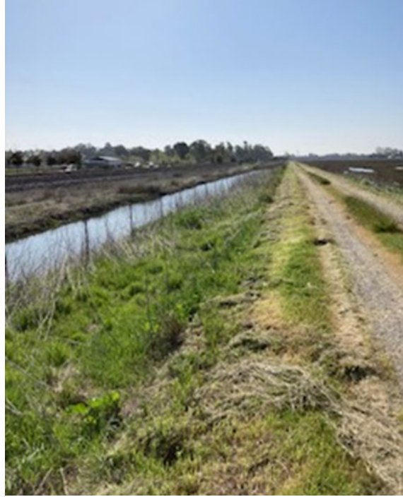
EBDA First Mile Horizontal Levee Project
