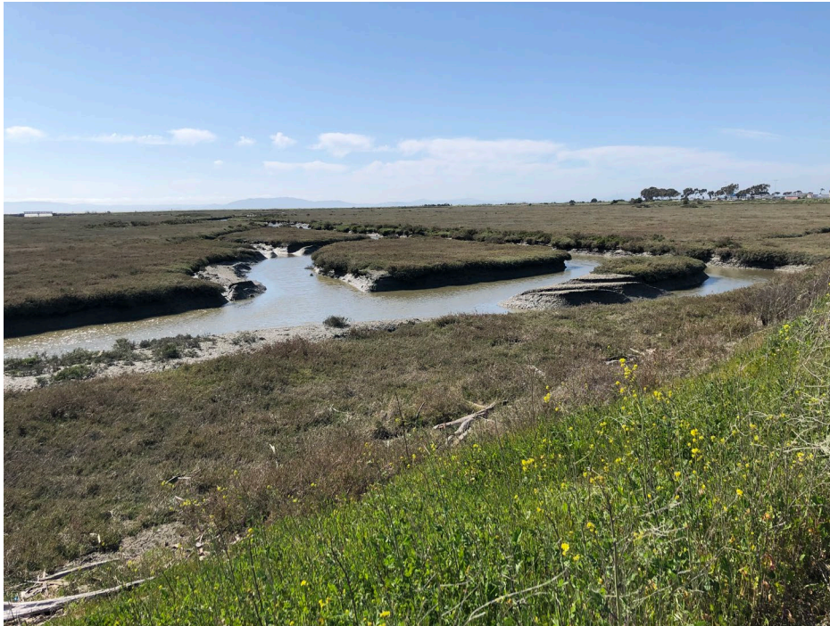
EBDA First Mile Horizontal Levee Project
