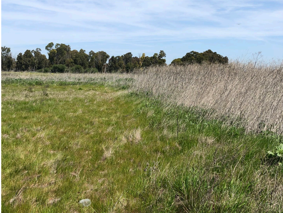
EBDA First Mile Horizontal Levee Project
