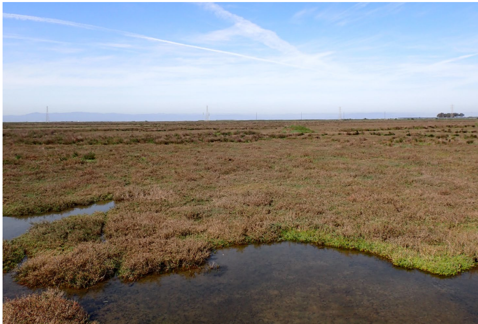
EBDA First Mile Horizontal Levee Project
