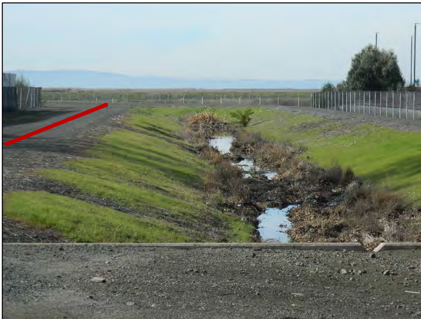
Photo 1 – View of drainage channel from Whitesell St. looking west. This channel was constructed after the EBDA pipeline, most likely resulting in locally reduced cover on the RCP force main. The EBRPD Construction Access Route will be on the south side berm of the drainage channel (photo left, red line). To photo right are the north side berm and railroad spur tracks.
