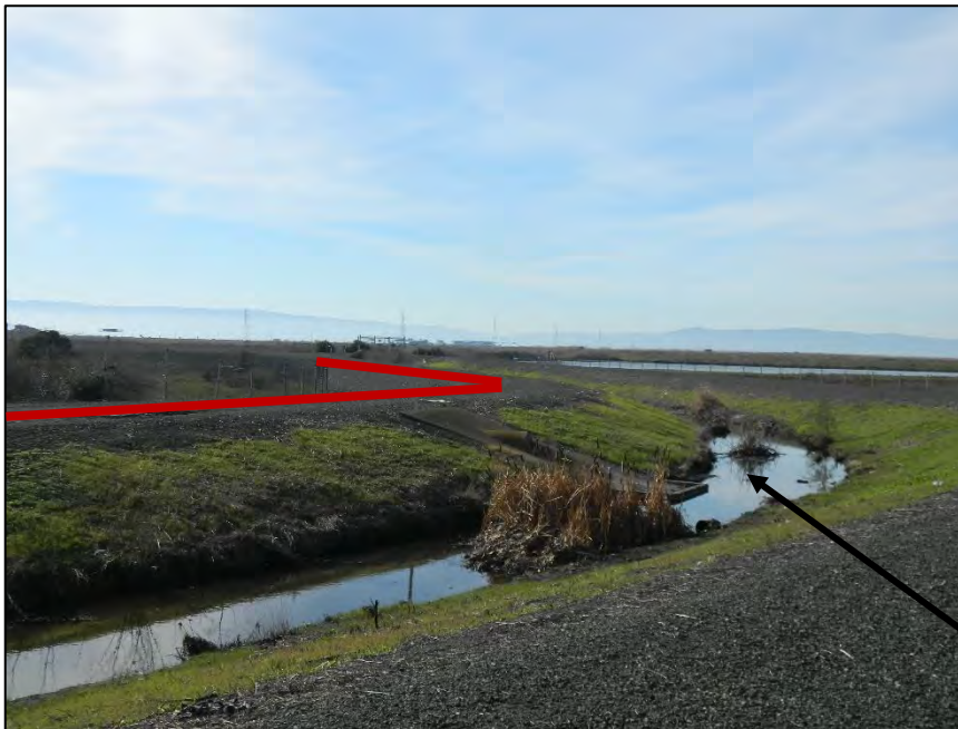
Photo 2 – View of drainage channel from railroad spur looking southwest. This channel was built after the EBDA pipeline, most likely resulting in locally reduced cover on the 60-inch RCP force main.
