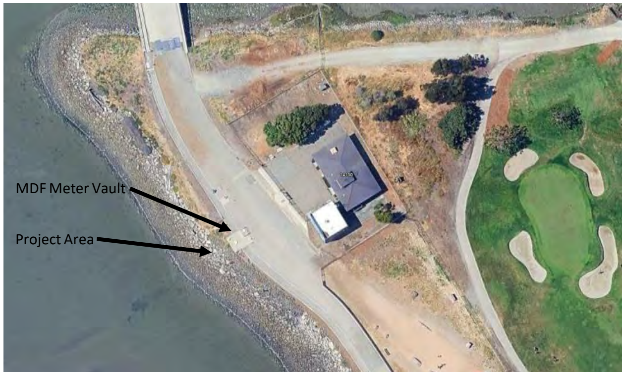
Marina Dechlorination Facility (MDF)
