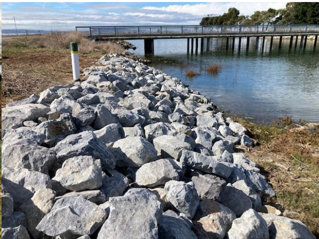
San Leandro Force Main – After
