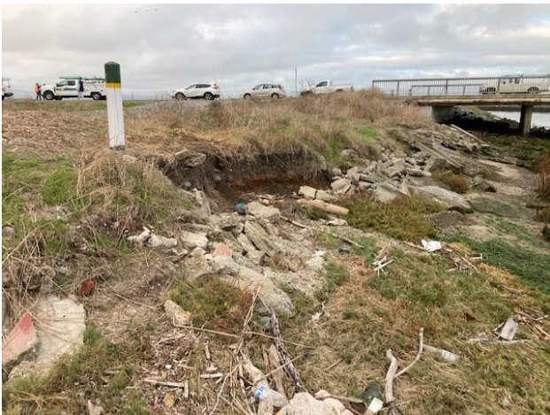
San Leandro Force Main – Before
