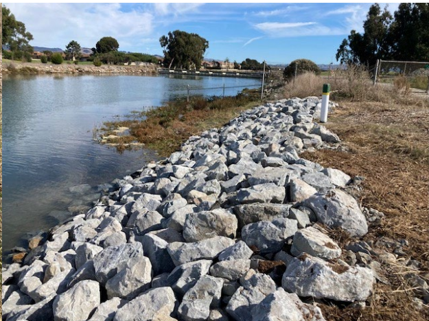
San Leandro Force Main – After
