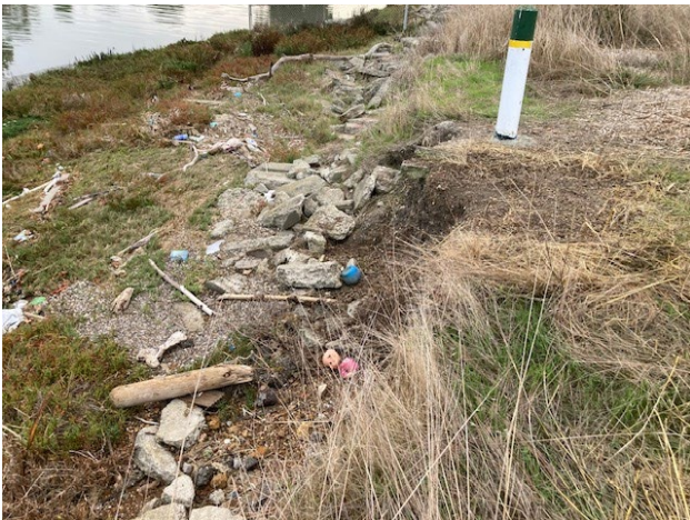
San Leandro Force Main – Before
