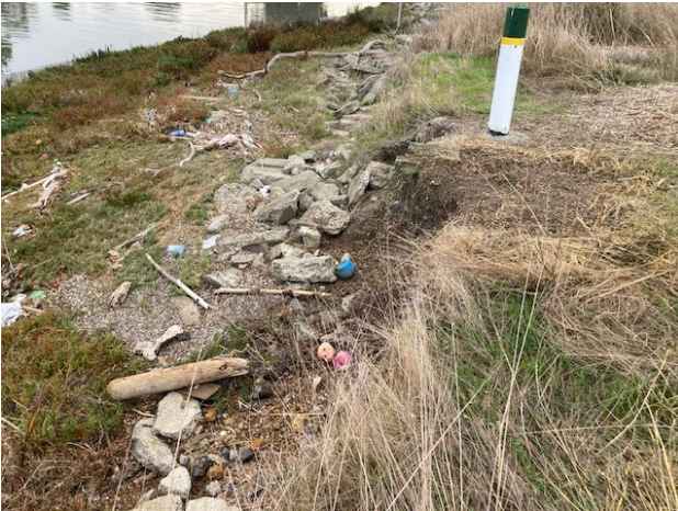
San Leandro Force Main – Before
