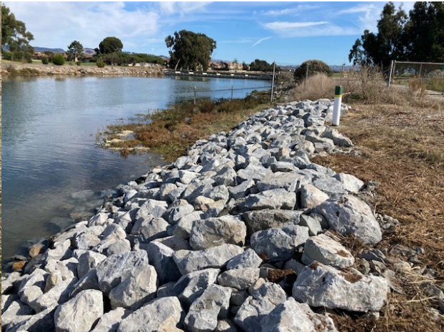
San Leandro Force Main – After
