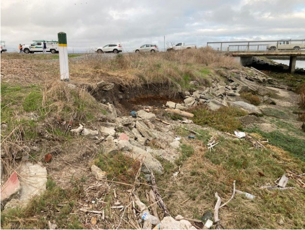
San Leandro Force Main – Before
