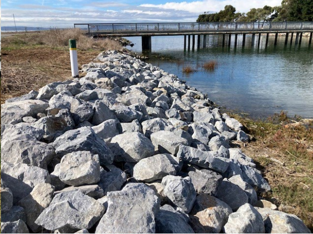
San Leandro Force Main – After
