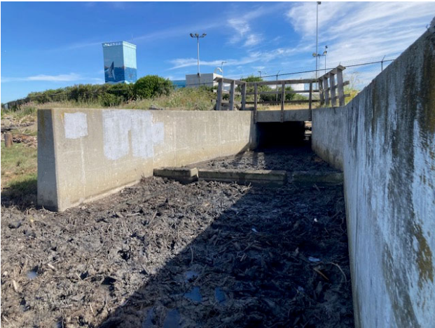
After Debris Removal
