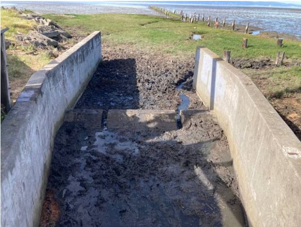
After Debris Removal
