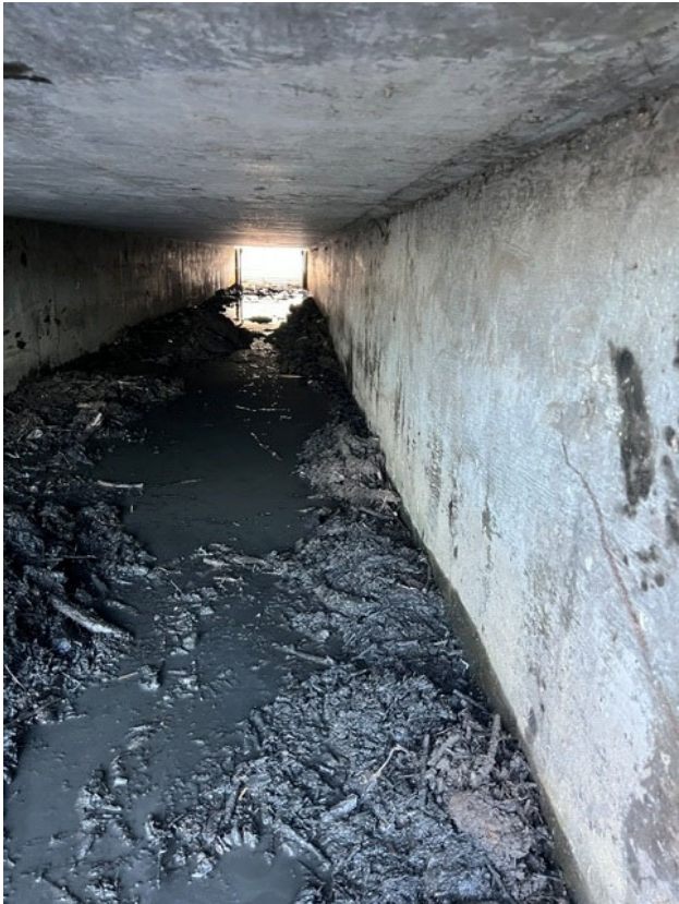
After Debris Removal
