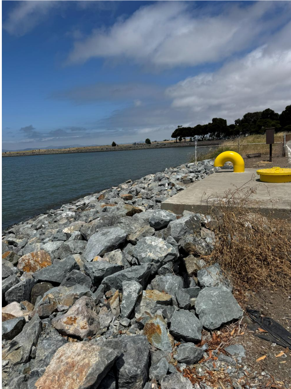
Figure 11. EBDA restored the rip rap on a 60-foot by 40-foot stretch of the levee along the Bay in front of the Marina Dechlorination Facility Meter Vault.
