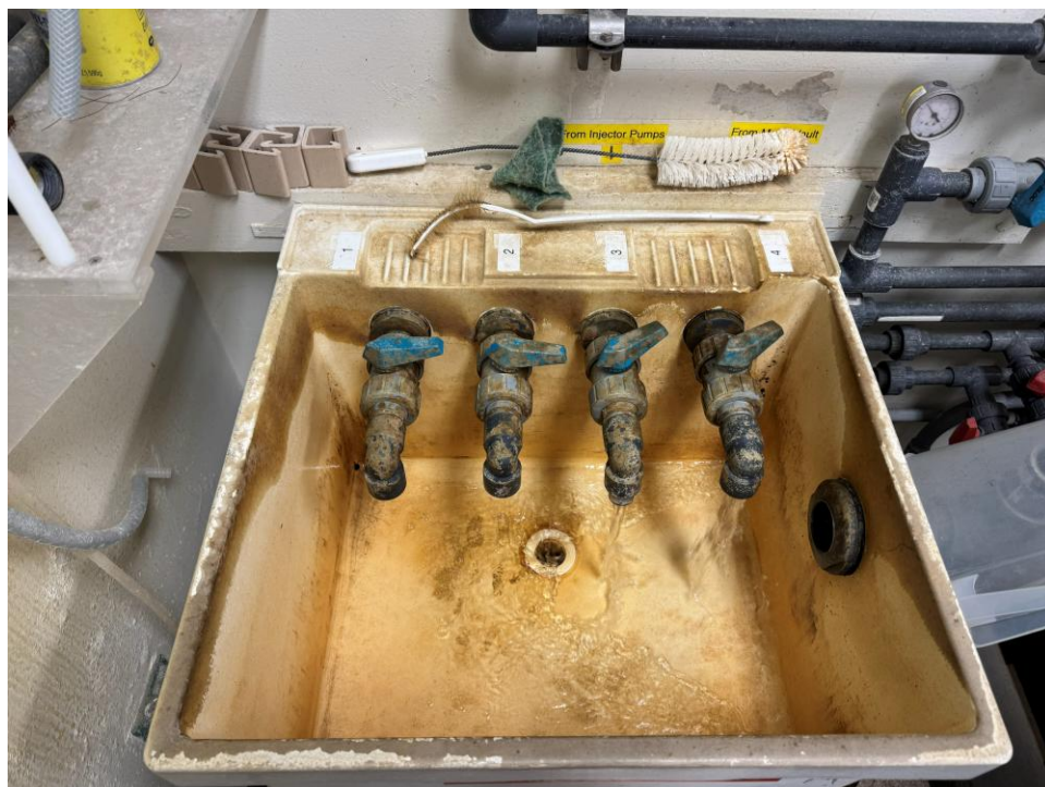
Figure 4. Influent and effluent sampling station.
